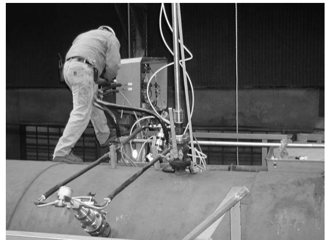
Verabar Model V550 installed
